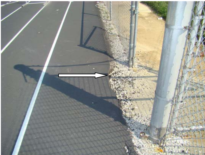
Picture #4 . . . shows the outside edges of the track that have having chunks to disappear.
