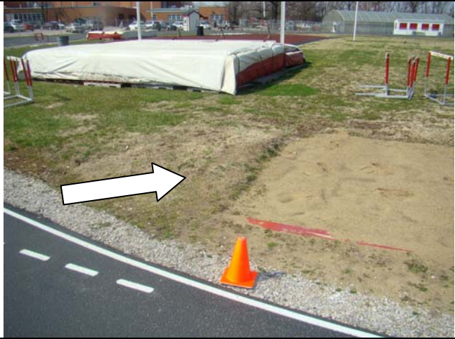
Picture #18 . . . the edges around the pit should all be ground level to help athletes avoid from tripping as they leave the pit.
