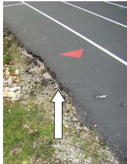
Picture #5 . . . show lane 8 with the edges of the track falling apart.
