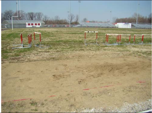
Picture #19 . . . Shows that you can not tell where the pit begins or ends.
