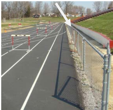
Picture #2 . . . shows the closeness of the fence to the athletes in lane 8, especially hurdlers with bad technique. Recommend capping this fence and the one on the backstretch and curve as well.
